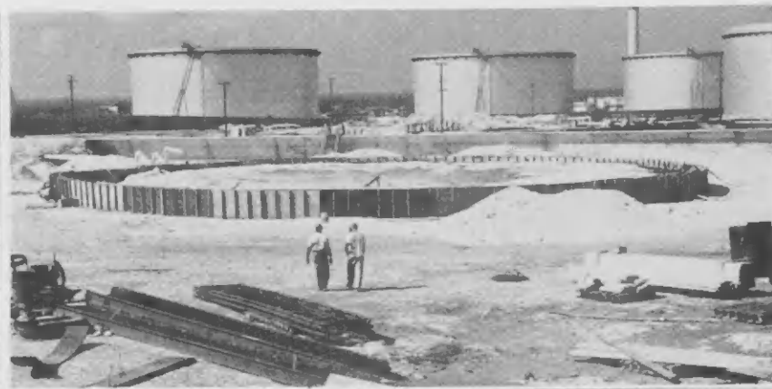
IN VARIOUS stages of construction in the tank farm are three huge gasoline storage tanks. The largest has a capacity of 80,000 barrels. All are floating-roof tanks. Because of special features incorporated in their design, the tanks can use a slightly thinner steel plating. New roof seals are more efficient in minimizing the evaporation of gasoline products.
